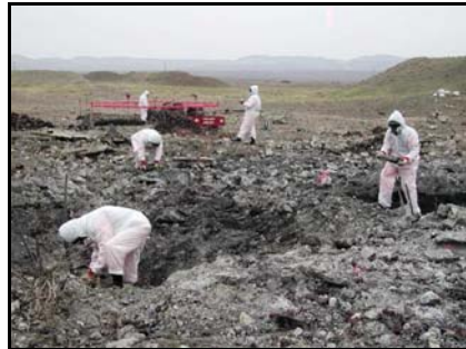
ANAMA personnel clearing a collapsed ammunition store – indicative of the problems at Saloglu
